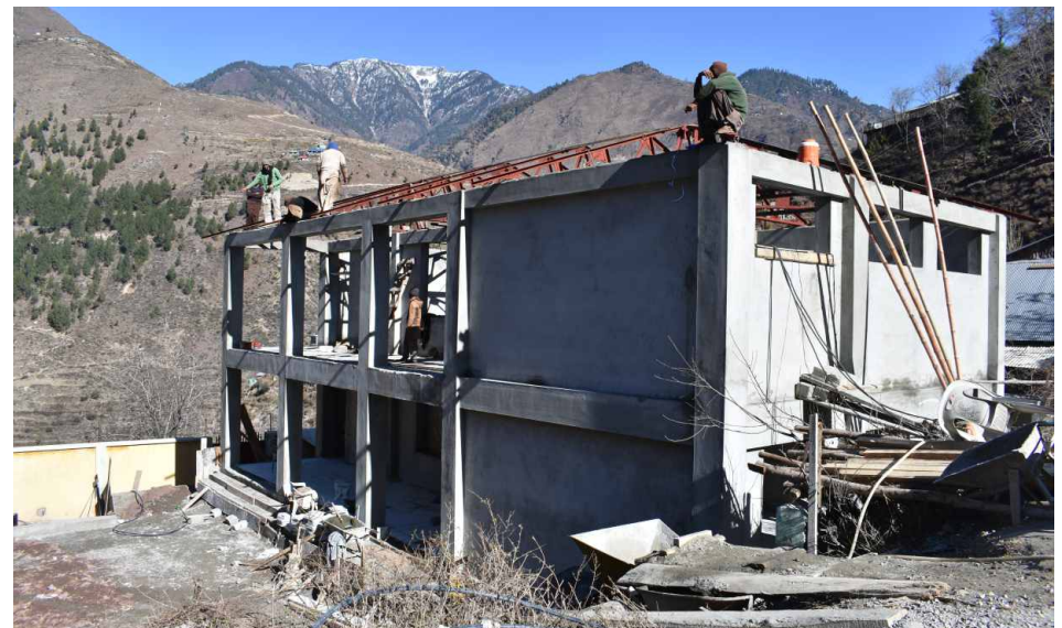
GPS Ratta Nalla UC Kawai Completed 67%
